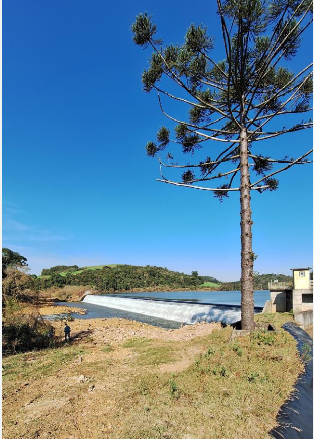
Image: Hydro Power Plant - Soledade
